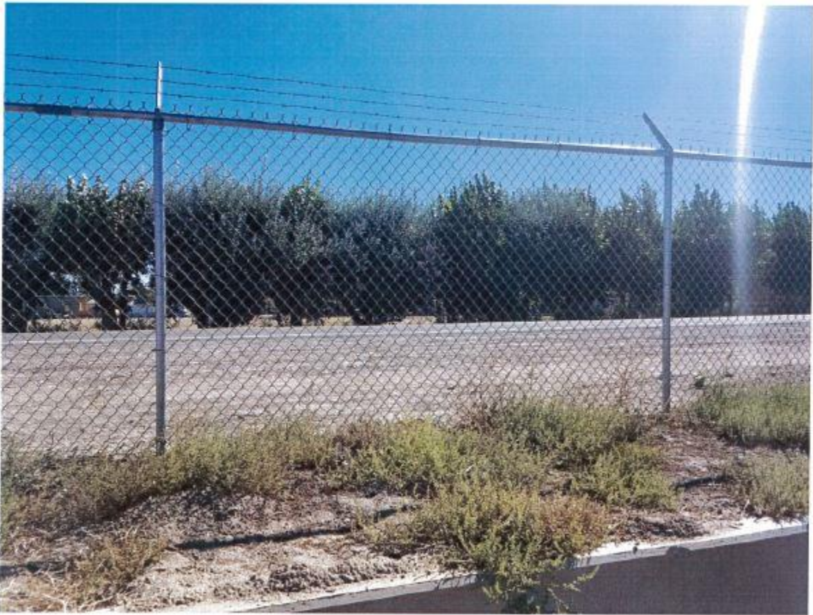
Existing airport fence
